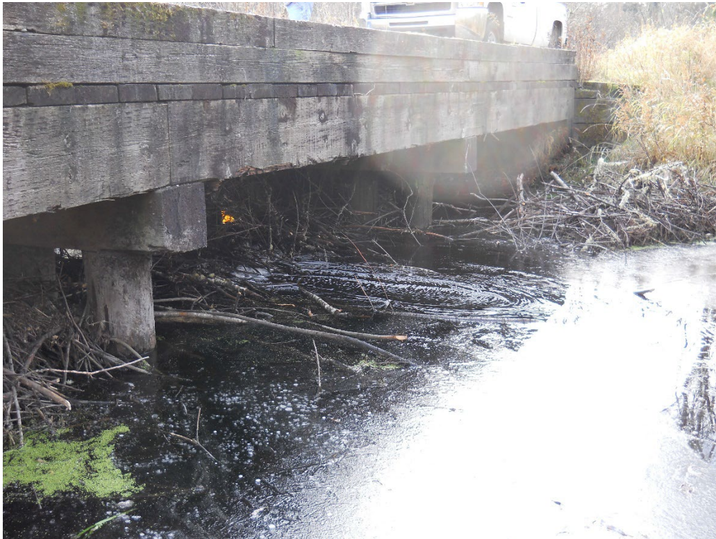
Beaver Dam beneath RR Trestle
