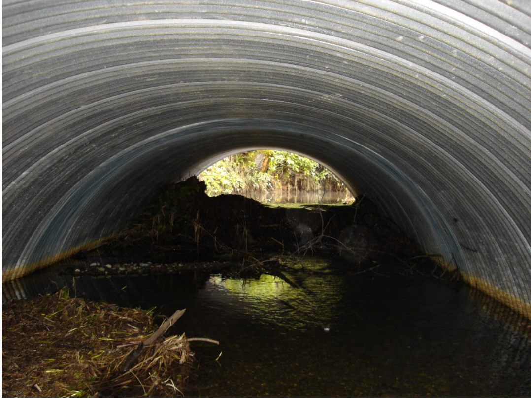
Looking upstream inside of a 6' diameter w/beaver dam
