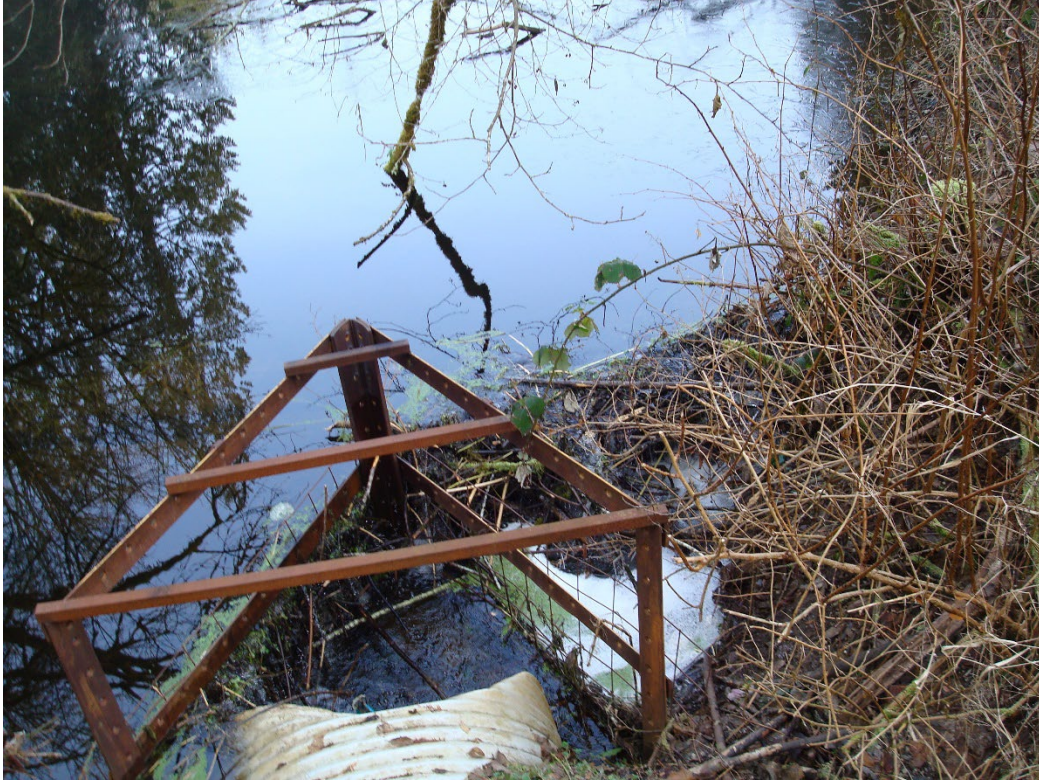
Deceivers help keep the dam from being built inside and is sized accordingly to fish species
