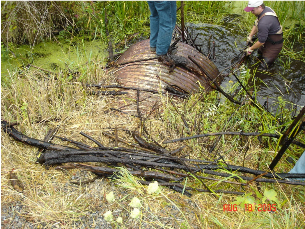
Beaver dam removal by hand – fortunately not much backwater
