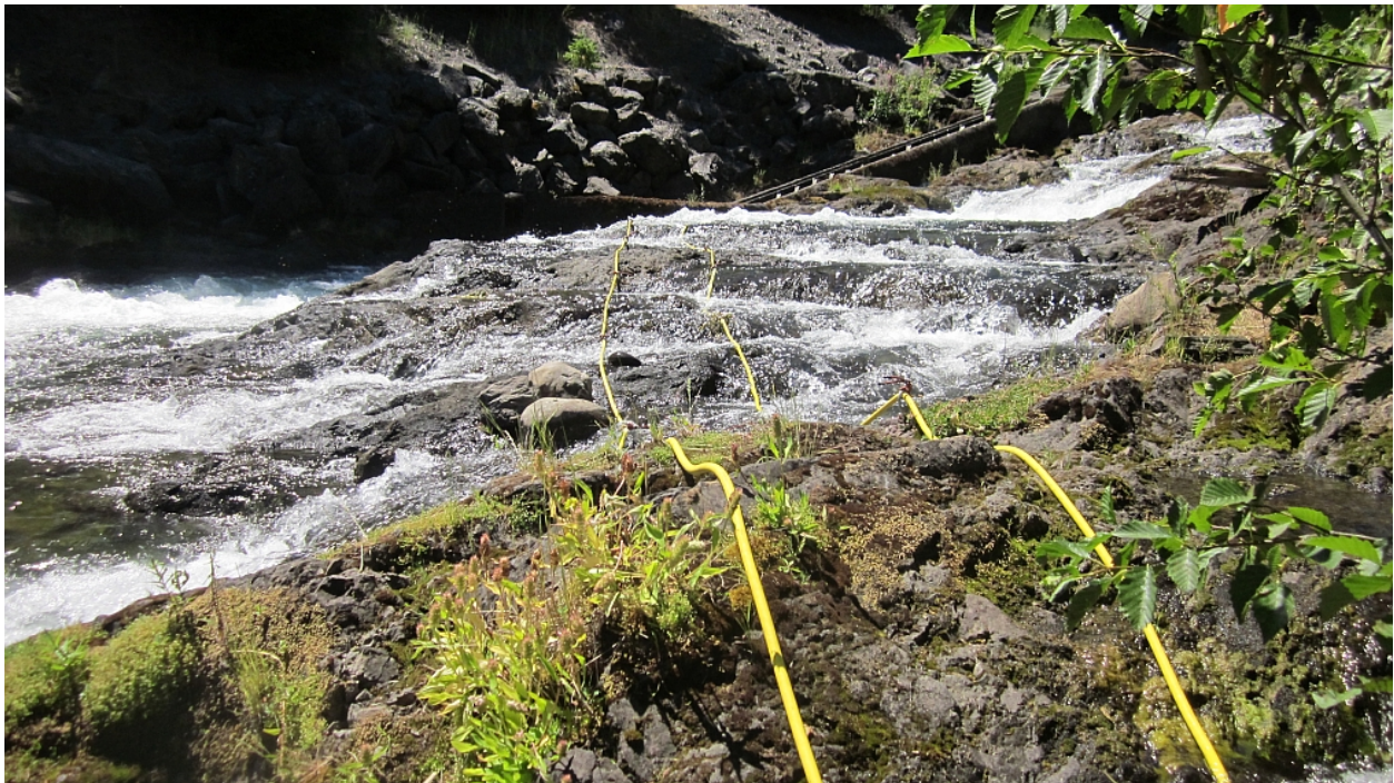
Figure 2. Antenna installed at the lower terminus of the spillway channel on July 9, 2013
