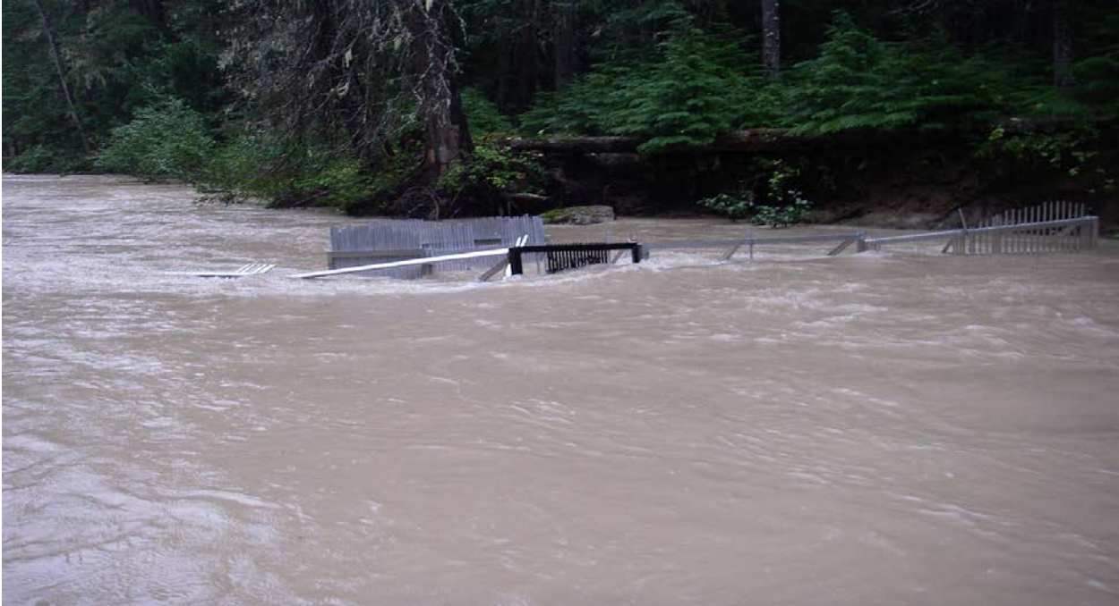
Figure 10. North Fork Tieton River fish trap during the high flow event which occurred at the end of September, 2013. This photo was taken the morning of September 29 th . The left weir panels have already washed downstream. The remaining panels and the box were gone soon after. The river continued to rise.
