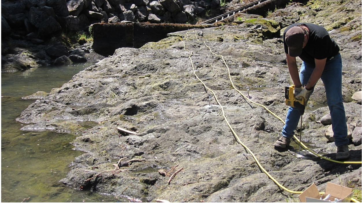
Figure 4. Installation of the lower spillway antenna on July 9, 2013
