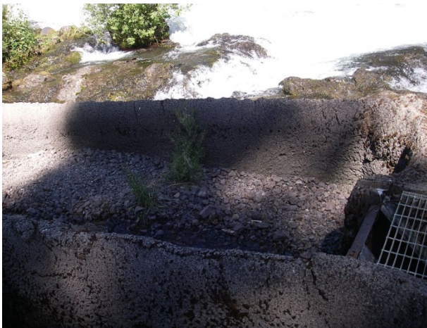
Totally dewatered downstream sections of the Denil ladder
