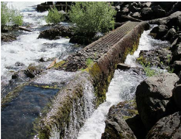
Upstream terminus of the Denil ladder completely clogged with bed load
