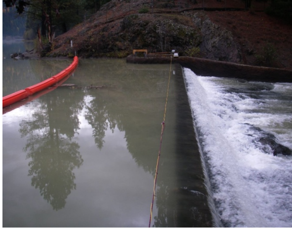
Antenna spanning the spillway weir
