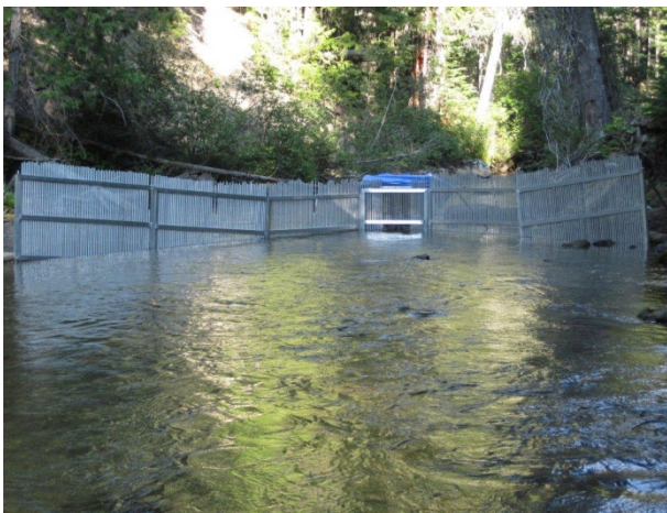
Completed picket-weir and box trap
