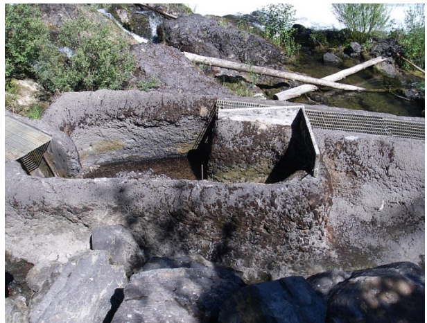
Upstream terminus of the Denil ladder completely clogged with bed load
