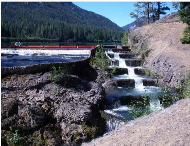
Pool-and-weir fish ladder in upper spillway channel
