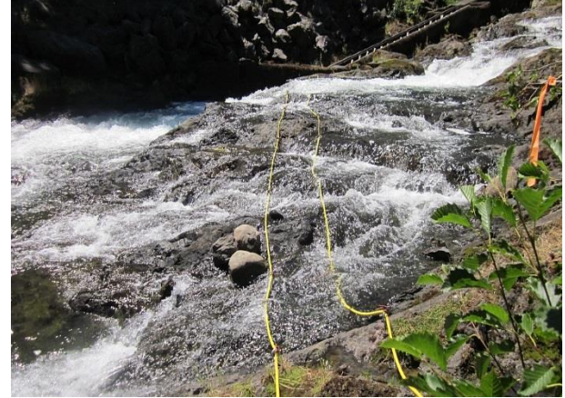
Lower spillway PIT tag detection antenna
