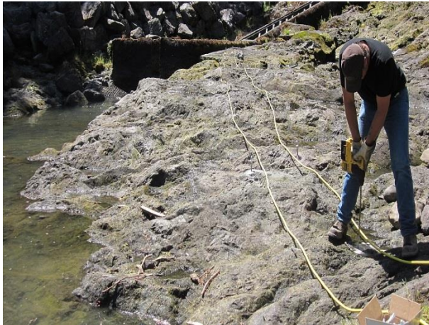
Drilling into bedrock on the lower spillway site
