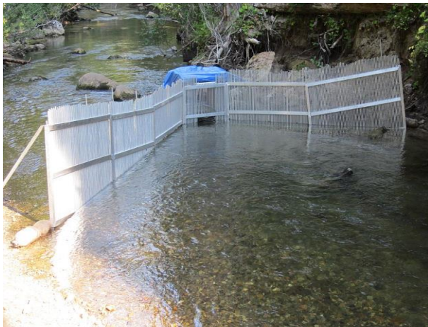
Completed picket-weir and box trap
