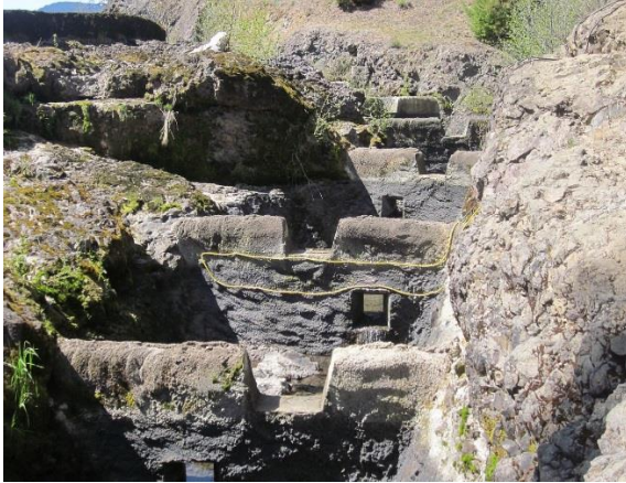
Lower ladder PIT tag detection antenna
