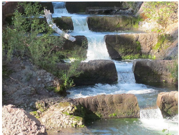
Pool-and-weir fish ladder in upper spillway channel
