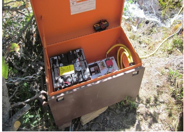
Batteries and readers kept inside locked job boxes
