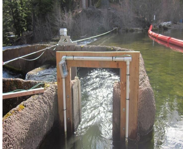
Upper ladder PIT tag detection antenna
