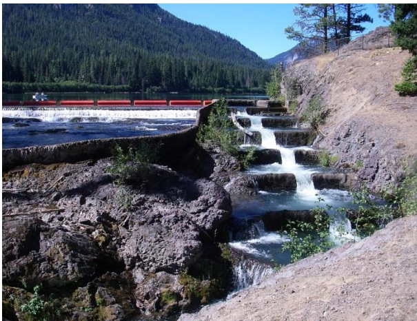
Pool-and-weir fish ladder in upper spillway channel
