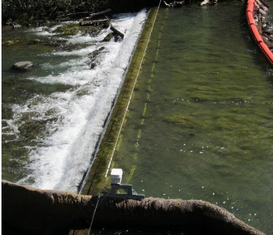
Upper spillway PIT tag detection antenna
