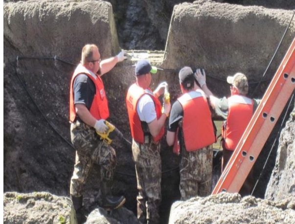
Installing the lower ladder antenna in 2014
