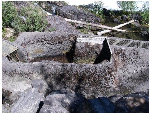
Totally dewatered downstream sections of the Denil ladder
