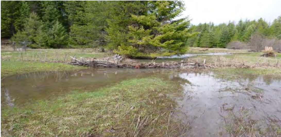
Figure 56. BDAs after peak flow constructed with posts driven into the streambed and woven with wicker weaves.
