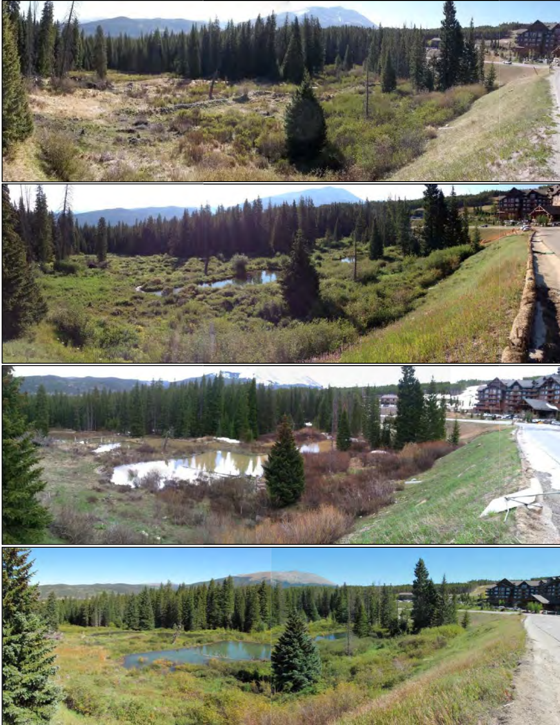
Figure 71: This series of photos shows a time lapse overview of a portion of the project area. Starting at the top, the photos are from (a) 2012 before the project, (b) 2013 after construction but before beavers arrived, (c) spring 2014 during runoff, and (d) summer 2014 after beavers significantly raised the height of dams.
