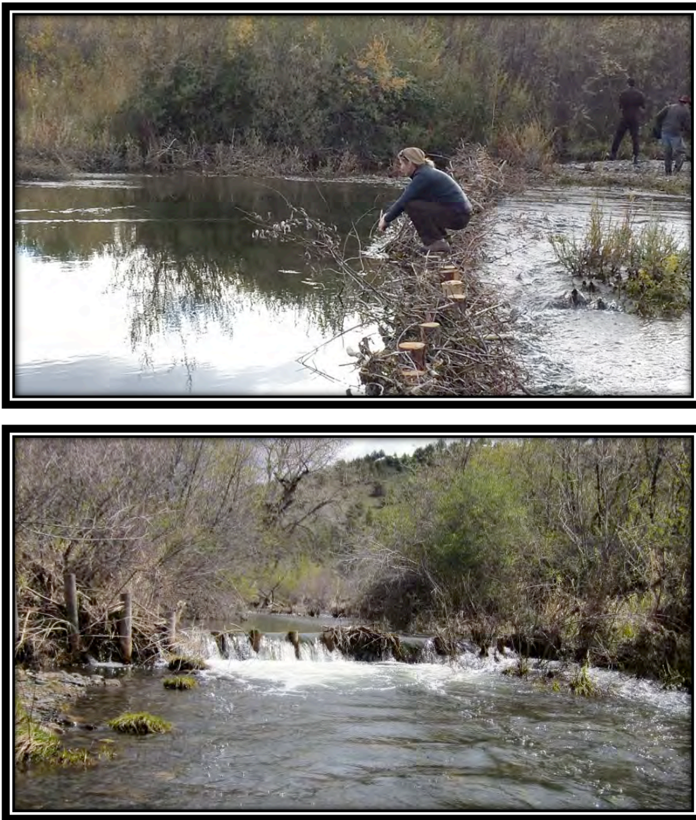
Figure 25: Examples of beaver dam analogues in Oregon and California.
