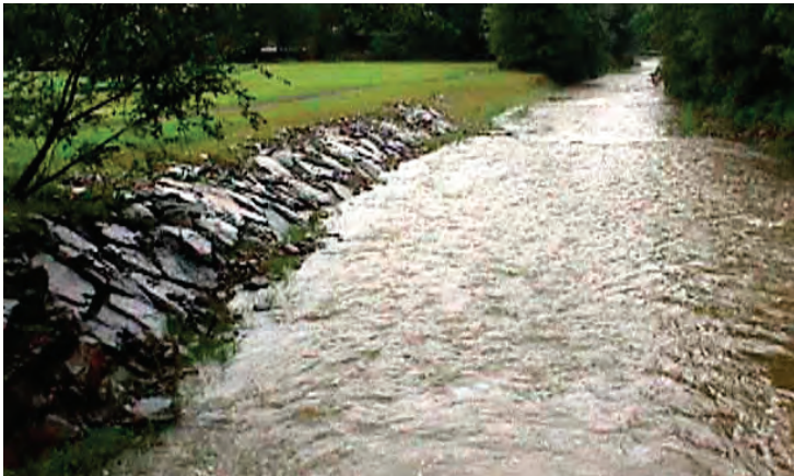
The most common technique for preventing streambank erosion is to protect the bank with rock riprap, but other streambank protection measures can be used as well. In this photograph, a retaining wall has also been used to protect a road. (Photograph by Mark Watts, Chemung County Soil and Water Conservation District.)
