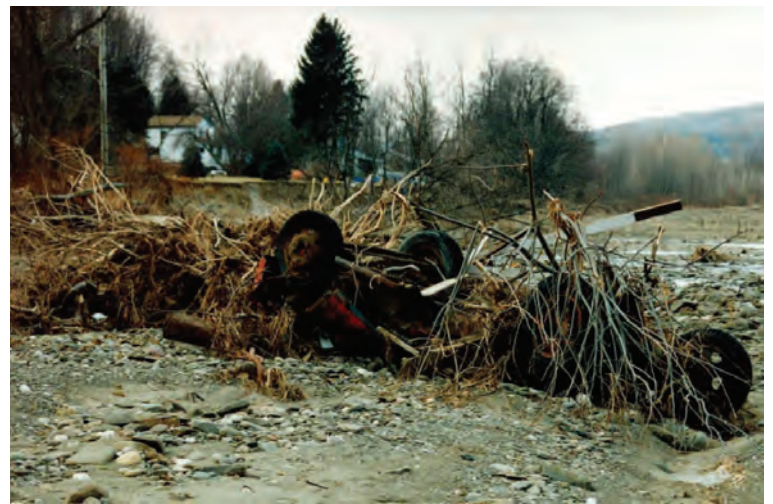
Streamside junk piles are ugly and ineffective bank protectors. They seldom stay in place during floods and frequently contain substances that cause water pollution. Even such massive items as automobiles and cement sidewalk slabs can be dislodged by the power of flowing water. Automobiles that were used to stabilize this stream in 1973 now wind up in the creek when the banks erode. (Photographs by Donald Lake, NYS Soil and Water Conservation Committee; and Mark Watts, Chemung County Soil and Water Conservation District.)
