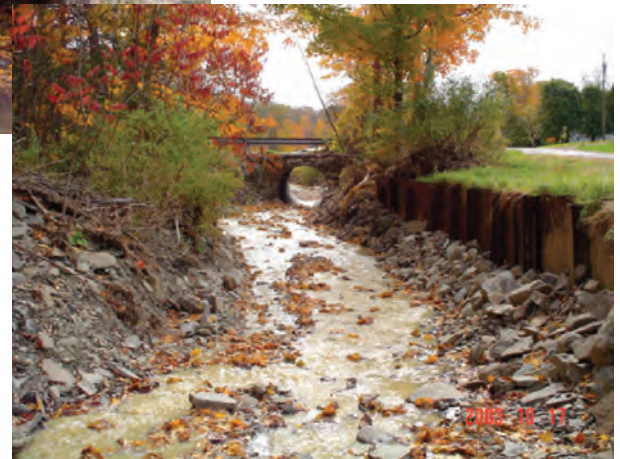
A narrow bridge or culvert restricts the stream channel and blocks flow on the floodplain. Improperly sized stream crossing structures can be a disaster waiting to happen and a money hole for maintenance. (Photographs by Mark Watts, Chemung County Soil and Water Conservation District.)
