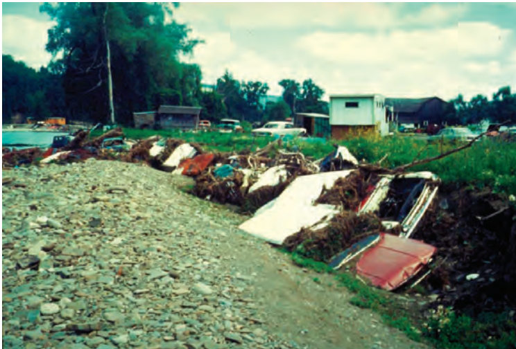
Streamside junk piles are ugly and ineffective bank protectors. They seldom stay in place during floods and frequently contain substances that cause water pollution. Even such massive items as automobiles and cement sidewalk slabs can be dislodged by the power of flowing water. Automobiles that were used to stabilize this stream in 1973 now wind up in the creek when the banks erode. (Photographs by Donald Lake, NYS Soil and Water Conservation Committee; and Mark Watts, Chemung County Soil and Water Conservation District.)
