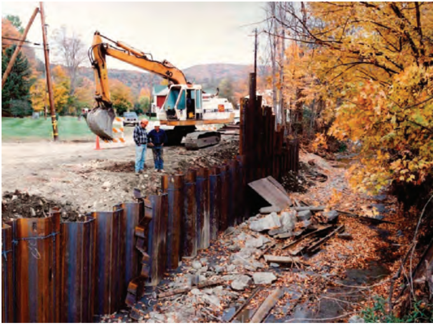
Sheet piling stabilization is a very expensive method of streambank protection and is sometimes only a temporary measure. Proper design is necessary to protect against erosion. (Photographs by Mark Watts, Chemung County Soil and Water Conservation District.)
