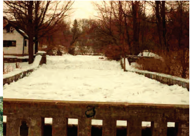
Confining flow to a paved channel may have flood conveyance benefits to the immediate area. However, habitat is lost and downstream areas will be impacted. (Photograph from “Stream Corridor Restoration: Principles, Processes, and Practices,” 10/98, by the Federal Interagency Stream Restoration Working Group.)
