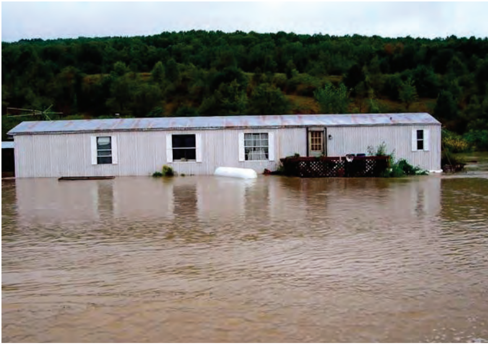
Inexpensive land in floodplains seems to attract mobile homes. If not properly anchored, a house can float off its foundation. Some have been swept far downstream. (Photograph courtesy of Steuben County Emergency Management Office.)
