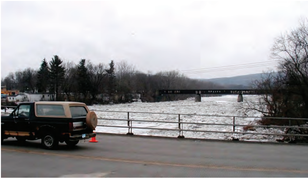
The constricted channel at a bridge may contribute to the formation of ice jams or debris piles. This ice jam was extensive enough to block flow in the river and flood surrounding areas. (Photograph courtesy of the Binghamton Forecast Office of the National Weather Service.)
