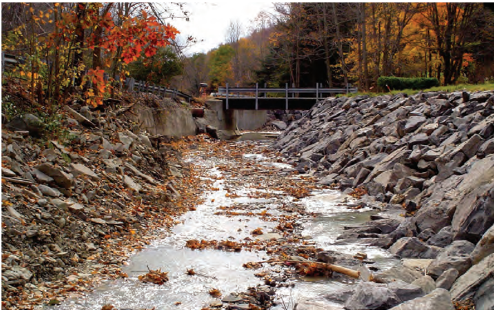
The most common technique for preventing streambank erosion is to protect the bank with rock riprap, but other streambank protection measures can be used as well. In this photograph, a retaining wall has also been used to protect a road. (Photograph by Mark Watts, Chemung County Soil and Water Conservation District.)
