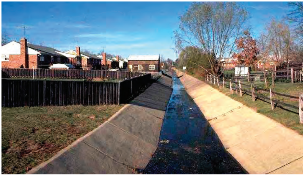
Confining flow to a paved channel may have flood conveyance benefits to the immediate area. However, habitat is lost and downstream areas will be impacted. (Photograph from “Stream Corridor Restoration: Principles, Processes, and Practices,” 10/98, by the Federal Interagency Stream Restoration Working Group.)
