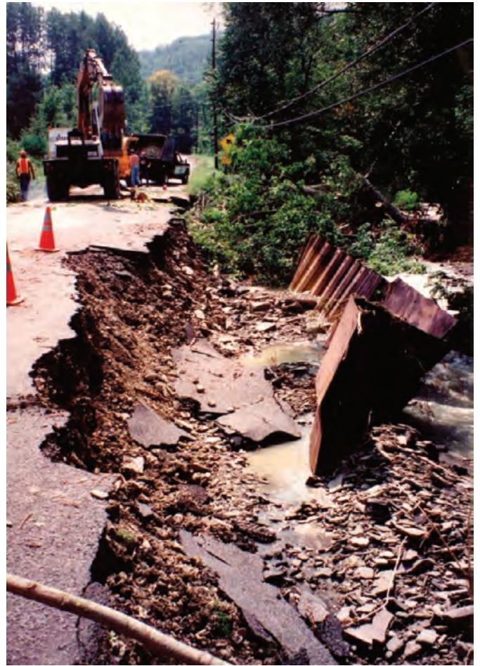
Sheet piling stabilization is a very expensive method of streambank protection and is sometimes only a temporary measure. Proper design is necessary to protect against erosion. (Photographs by Mark Watts, Chemung County Soil and Water Conservation District.)
