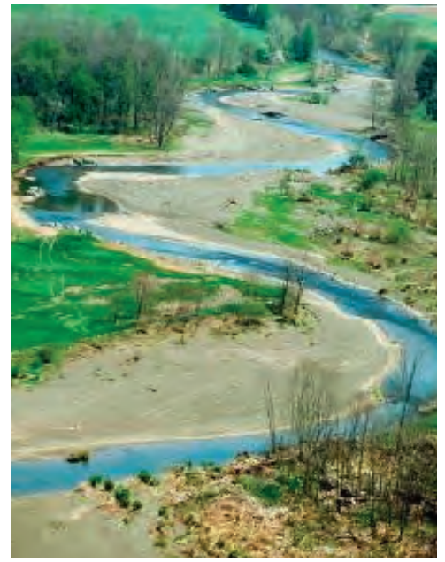
The shape and location of this stream channel has been re-built based on “natural stream design” principles. The objective is to create a stream channel in which the energy is balanced. (Photograph courtesy of Greene County Soil and Water Conservation District.)
