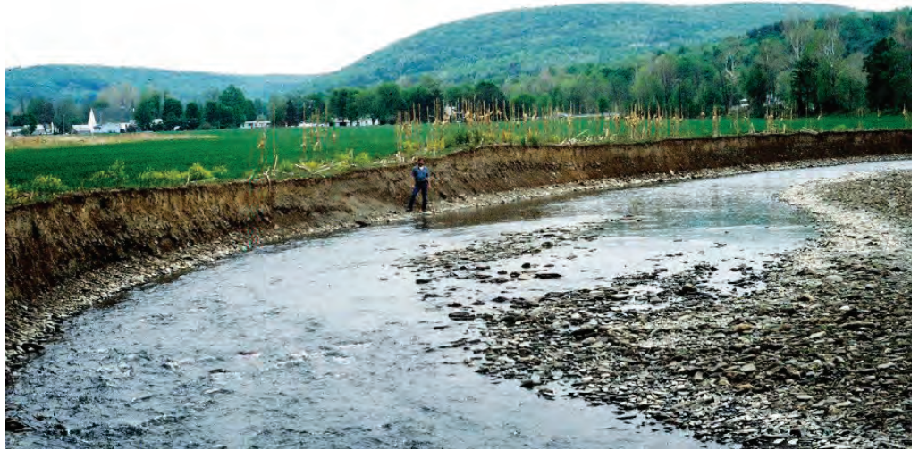
Bentley Creek washed out 4 ½ acres of cornfield in a single storm event. (Photograph by Mike Lovegreen, Bradford County Conservation District.)
