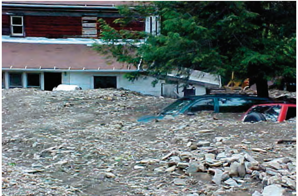
Flash flooding of a small stream piled gravel up to four feet deep on the floodplain. The best protection against this damage would have been to locate development away from the stream on high ground. (Photograph courtesy of Steuben County Emergency Management Office.)
