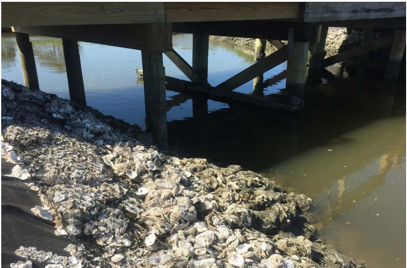
Tidal crossing incorporating bagged oyster shells for bank stabilization on Little St. Simons Island. Credit: Sara Gottlieb/TNC
