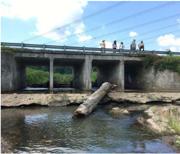
Before: 2016 photo of a multibox culvert with an impassible lip and flow underneath the structure on Raccoon Creek at Raccoon Creek Road, Paulding County. Credit: Katie Owens/TNC
