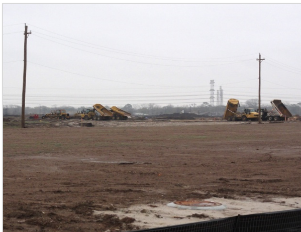
Figure 10. Land-leveling in a new subdivision. League City, TX.
