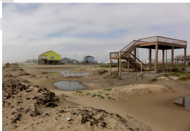
Figure 5. Beach damage and flooded blowouts from Hurricane Ike. Bolivar Peninsula.
