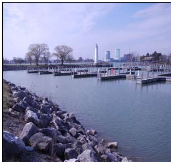
Milliken State Park marina in the Detroit River including riprap that extends into the nearshore habitat.
