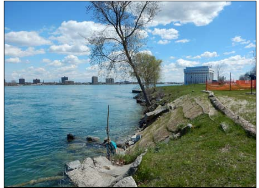
Kiefer Park shoreline following restoration efforts.
