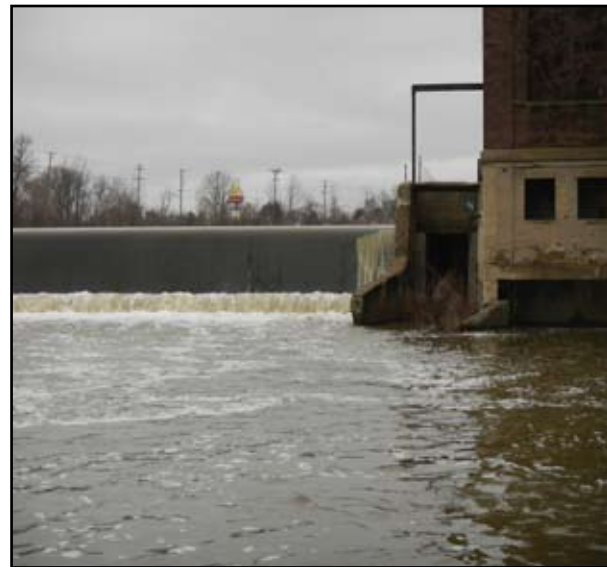
Peninsular Park Hyrdoelectric Structure
