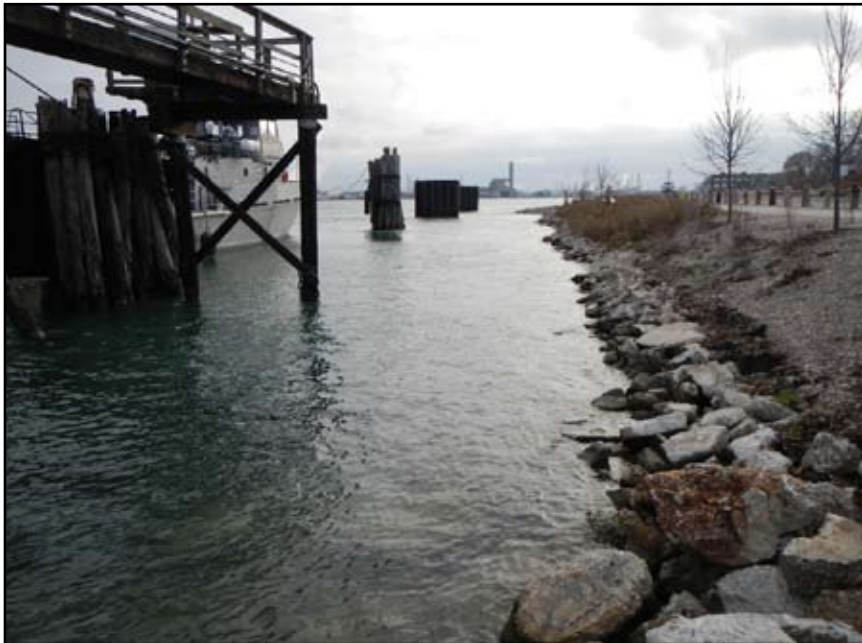
Blue Water River Walk restoration site in Port Huron.
