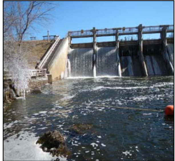
Sample location downstream of the Barton Dam in Ann Arbor.
