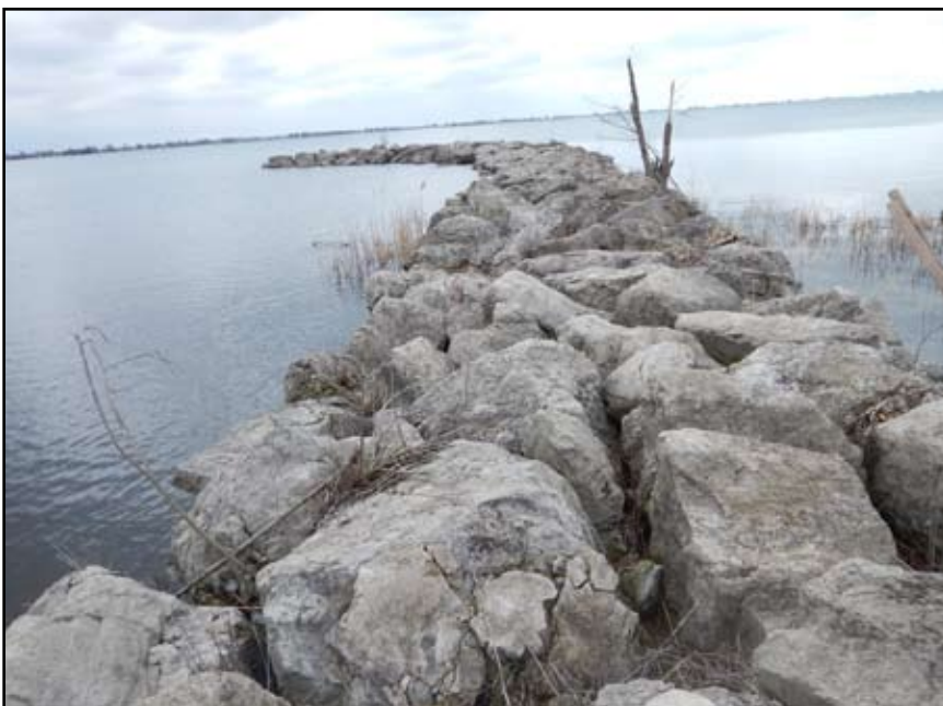
Riprap dyke located at the Fairhaven boat launch.
