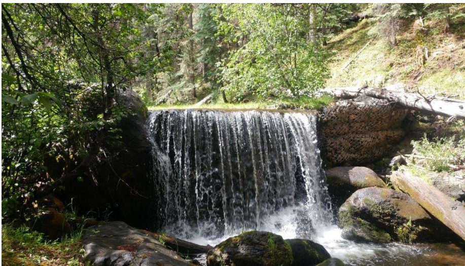
Protective gabion barrier on Paradise Creek, Arizona.
