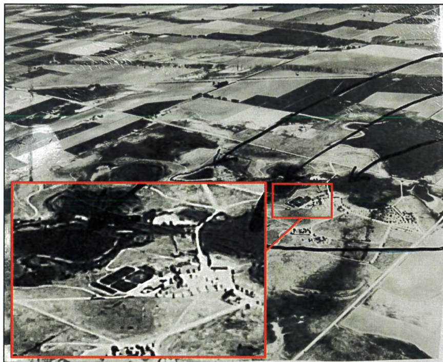
Figure 1. Aerial view of the Dexter Federal Fish Hatchery before 1950 showing the original configuration of Ponds A-D. 1960 Annual Report caption “Station before 1950.”
