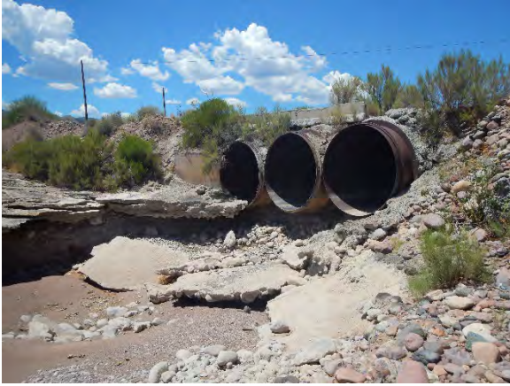
Photo 20. View of culvert system that is a barrier to upstream fish passage at East del Chi Dr crossing, 7/28/20. Each culvert is approximately 6 ft in diameter.
