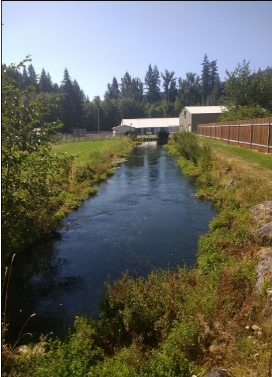
Figure 2. Sampling Unit 1: hatchery intake channel.
