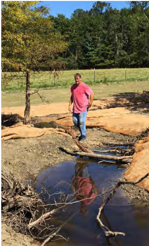
Chipola River tributary in Marianna, Florida. Restored meander geometry to channelized tributary to benefit listed mussels, credit USFWS/Chris Metcalf.
