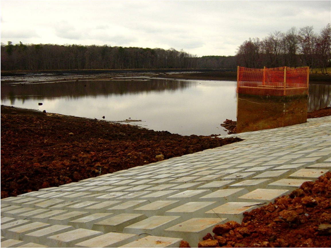
Construction at Patuxent Research Refuge
