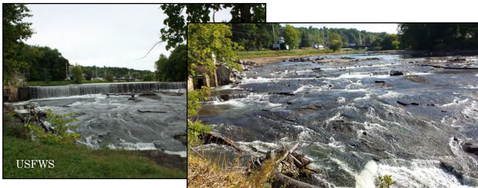
Boquet River before and after removal of Willsboro Dam in Willsboro, NY
