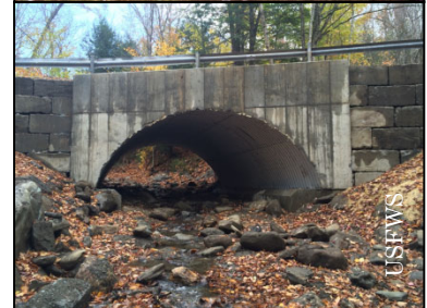
Restoring natural stream flow and fish passage under a road
