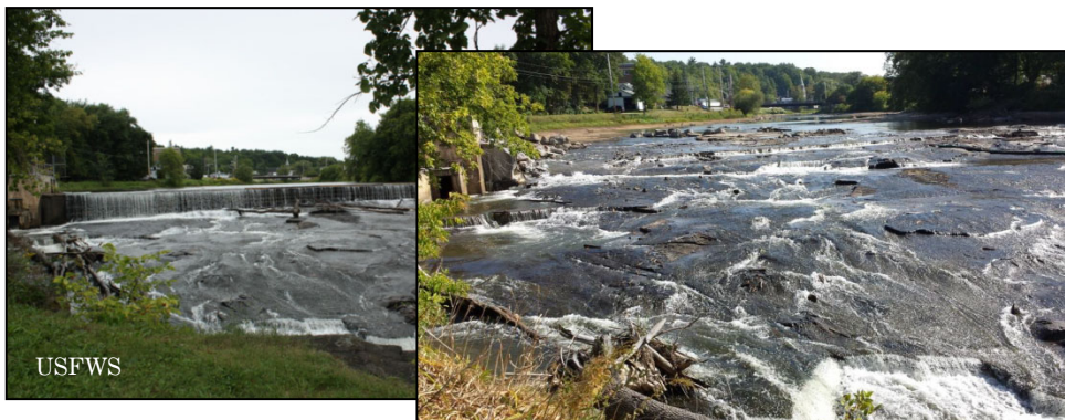
Bouquet River before and after removal of Willsboro Dam in Willsboro, NY
