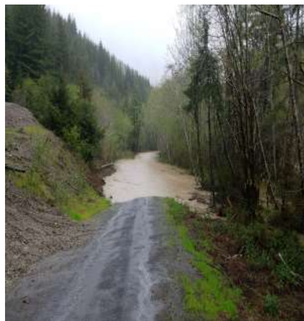
Top: Relocated road (left) and the restored side channel and floodplain habitat (center) after project implementation.
