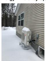
In an effort to reduce fossil fuel consumption and improve the efficiency of the refuge's infrastructure, an electric mini-split heat pump and hybrid electric hot water heater were installed at the Nulhegan Basin crew quarters. The two high efficiency electric units will dramatically reduce the refuge's reliance on fuel oil and reduce the operating costs associated with heating the crew quarters.
