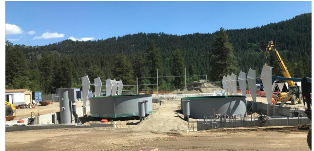
Figure 8: New circular tank systems will come with new stressors including water quality and water speed. If these stressors are not carefully managed, they will contribute to disease risk.
