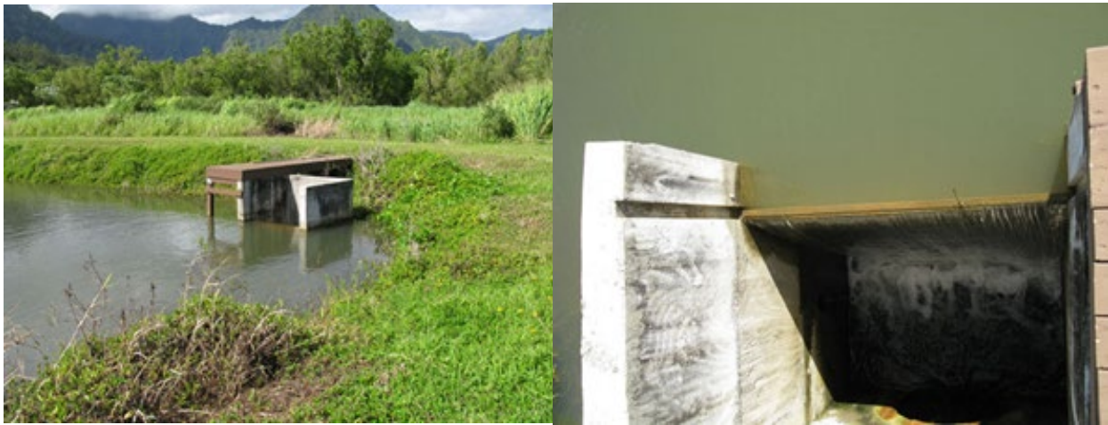
Cement drain boxes with wooden slats inserted and grooved boards are used to control water levels.
