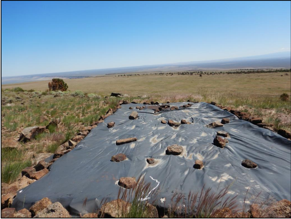
Figure H-7. Guzzler apron that catches water and directs it to storage tanks on Hart Mountain NAR.
