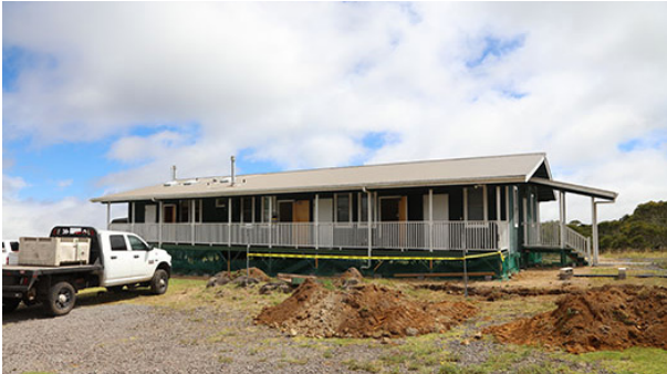
Staff Residence Bunkhouse
