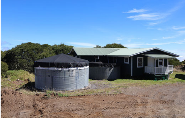
Existing Volunteer Bunkhouse
