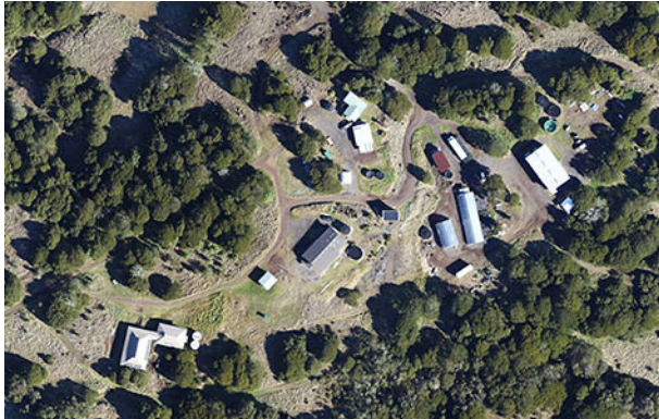
Existing Station Aerial
