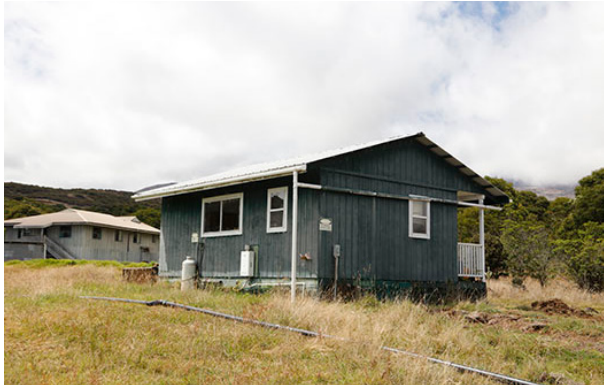
Existing BRD Cabin
