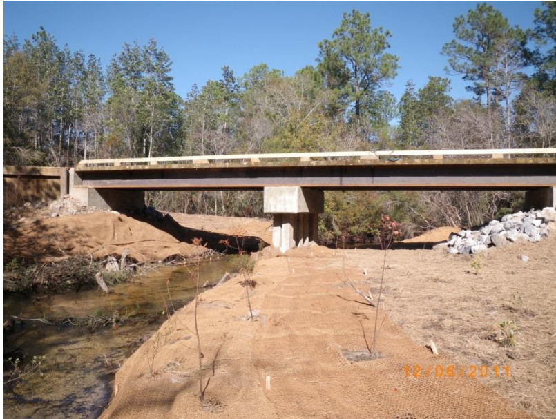
Figure 3. Bridge with Floodplain and Height Capacity for 100 yr Flows.
