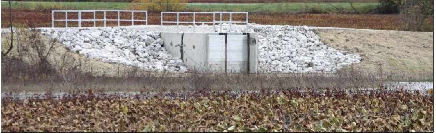
A water structure at Pool 2B can be open and closed, allowing for fish to move through. USFWS
