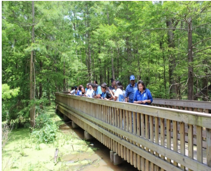
Visitor Facility enhancements include structures such as hunting blinds, fishing piers, observation decks, and boardwalks such as this one at Anahuac Refuge (Texas).
