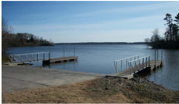
Crab Orchard NWR West End boat ramp and docks improvement project.
