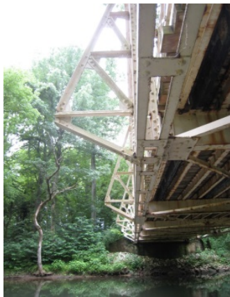
Figure 1. Duvall Bridge prior to restoration.
