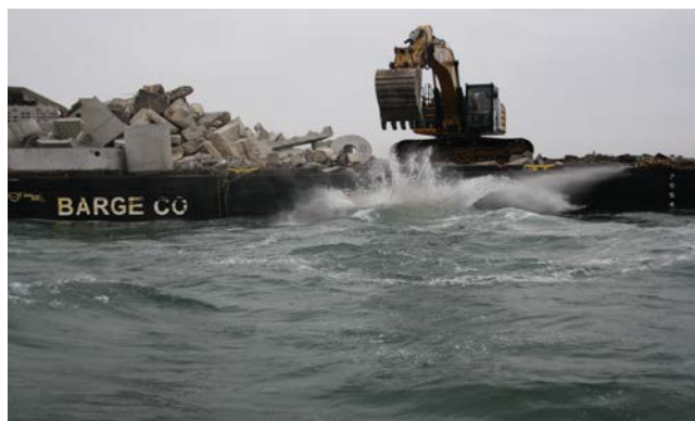
Dumping debris to create an artificial reef. Credit: Massachusetts Division of Marine Fisheries
