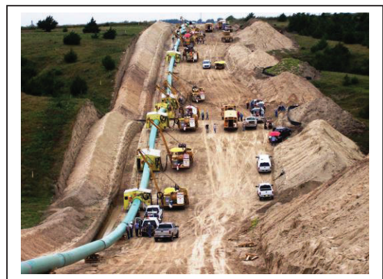
Figure 2.0-1 – Leveled work corridor for pipeline installation, showing cut hillsides and evident dewatering into the pipeline trench. Heavy equipment and pick-up trucks provide a scale.
