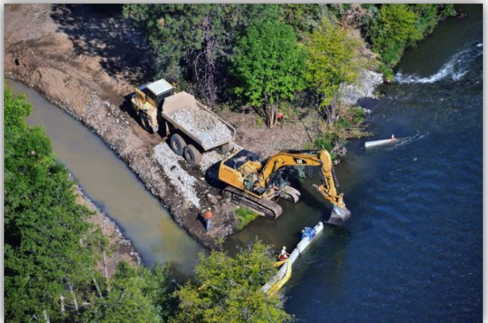
Channel Rehabilitation at Bucktail 2016. Credit: Kenneth DeCamp
