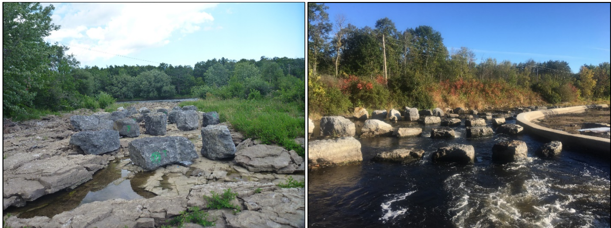
Nature-like fishway at the Eel Weir development (during construction and after)
