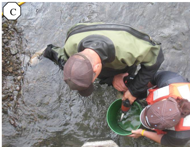
Figure 2. Pictures of White Salmon Working Group members installing the 4 inch angle iron and drilling into the concrete sill at the White Salmon Ponds at river mile 1.4. (A) Angle iron was installed to shield the cable that holds the resistance board weir in place and extended the entire wetted width of the White Salmon River on the existing concrete sill. (B) Angle iron was placed immediately behind the submerged pieces of the historical White Salmon Weir. (C, D) U.S. Fish and Wildlife Service personnel drilling in concrete for installation of eyebolts to hold the submerged cabling.
