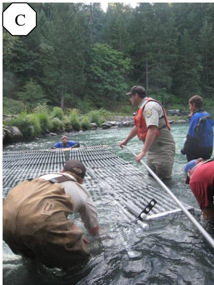
Figure 3. Installation of resistance board weir panels adjacent to the White Salmon Ponds at river mile 1.4 on August 20 th , 2009. Prefabricated panels were floated in the river (A) pulled by rope into position for attachment (B) and a connecting pipe (C) was threaded between two panels by personnel positioned at the end of the weir (D) and connected throughout the length of the panel (E). On August 20 th , the installation of panels required 14 people and was completed in approximately 3.5 hours and included installation of a video passage system.
