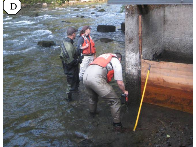
Figure 2. Pictures of White Salmon Working Group members installing the 4 inch angle iron and drilling into the concrete sill at the White Salmon Ponds at river mile 1.4. (A) Angle iron was installed to shield the cable that holds the resistance board weir in place and extended the entire wetted width of the White Salmon River on the existing concrete sill. (B) Angle iron was placed immediately behind the submerged pieces of the historical White Salmon Weir. (C, D) U.S. Fish and Wildlife Service personnel drilling in concrete for installation of eyebolts to hold the submerged cabling.
