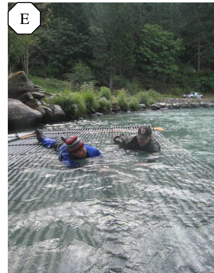
Figure 3. Installation of resistance board weir panels adjacent to the White Salmon Ponds at river mile 1.4 on August 20 th , 2009. Prefabricated panels were floated in the river (A) pulled by rope into position for attachment (B) and a connecting pipe (C) was threaded between two panels by personnel positioned at the end of the weir (D) and connected throughout the length of the panel (E). On August 20 th , the installation of panels required 14 people and was completed in approximately 3.5 hours and included installation of a video passage system.
