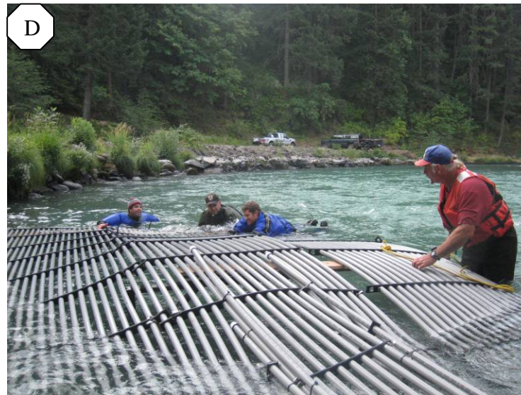
Figure 3. Installation of resistance board weir panels adjacent to the White Salmon Ponds at river mile 1.4 on August 20 th , 2009. Prefabricated panels were floated in the river (A) pulled by rope into position for attachment (B) and a connecting pipe (C) was threaded between two panels by personnel positioned at the end of the weir (D) and connected throughout the length of the panel (E). On August 20 th , the installation of panels required 14 people and was completed in approximately 3.5 hours and included installation of a video passage system.
