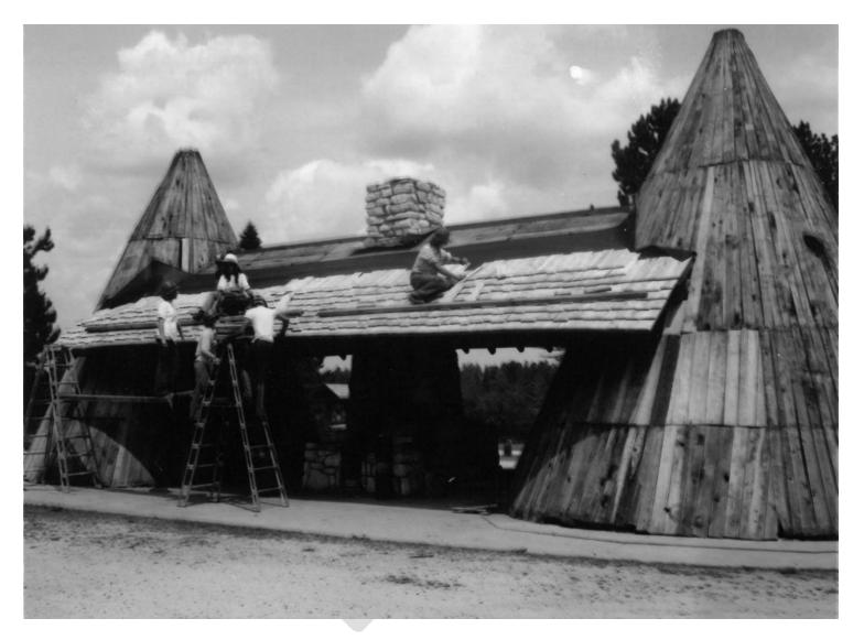
Photo 5: The Show Pool Shelter in 1974 when it was being covered with cedar shakes for the first time.
