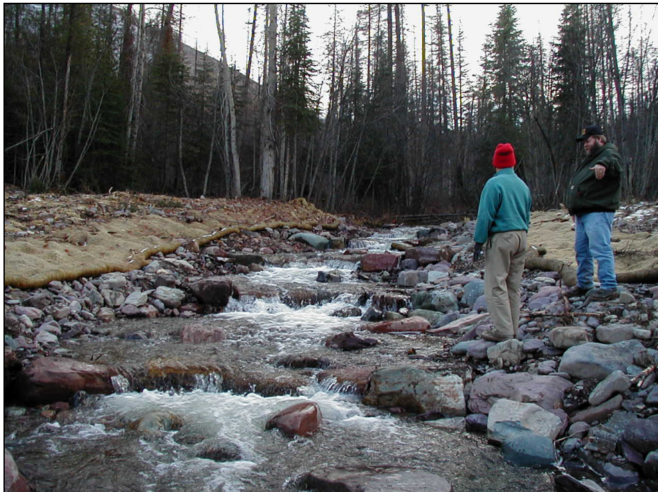
Lookout Creek during implementation. Note vortex weirs that provide grade control through the restored reach.
