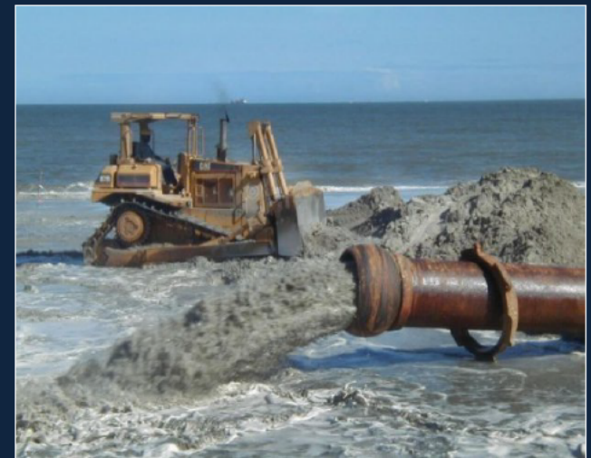
Beach nourishment on Tybee Island, Georgia (2008, U.S. Army Corps of Engineers)
