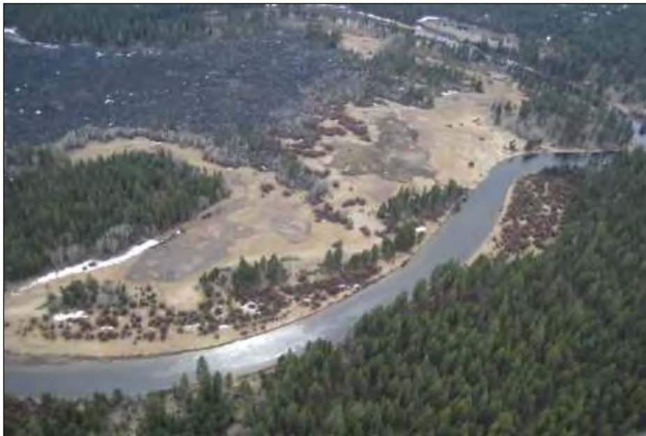
Figure 53. Aerial photo of East Slough Camp complex on March 18, 2016 with flows at WICO of 28 cfs and BENO at 744 cfs.
