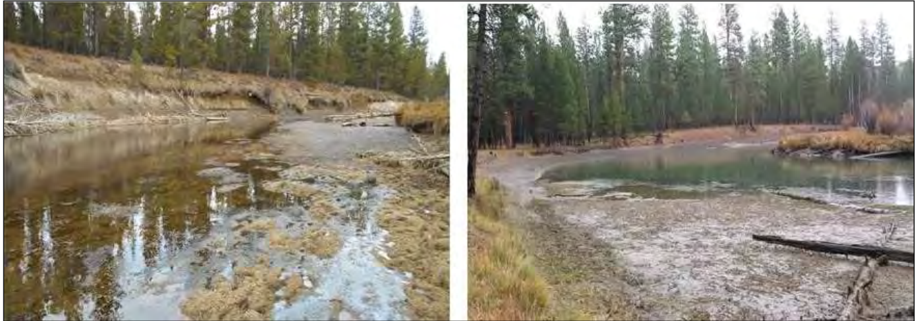
Figure 24. Photos of the Deschutes River channel condition during low winter flows from Wickiup Dam.
