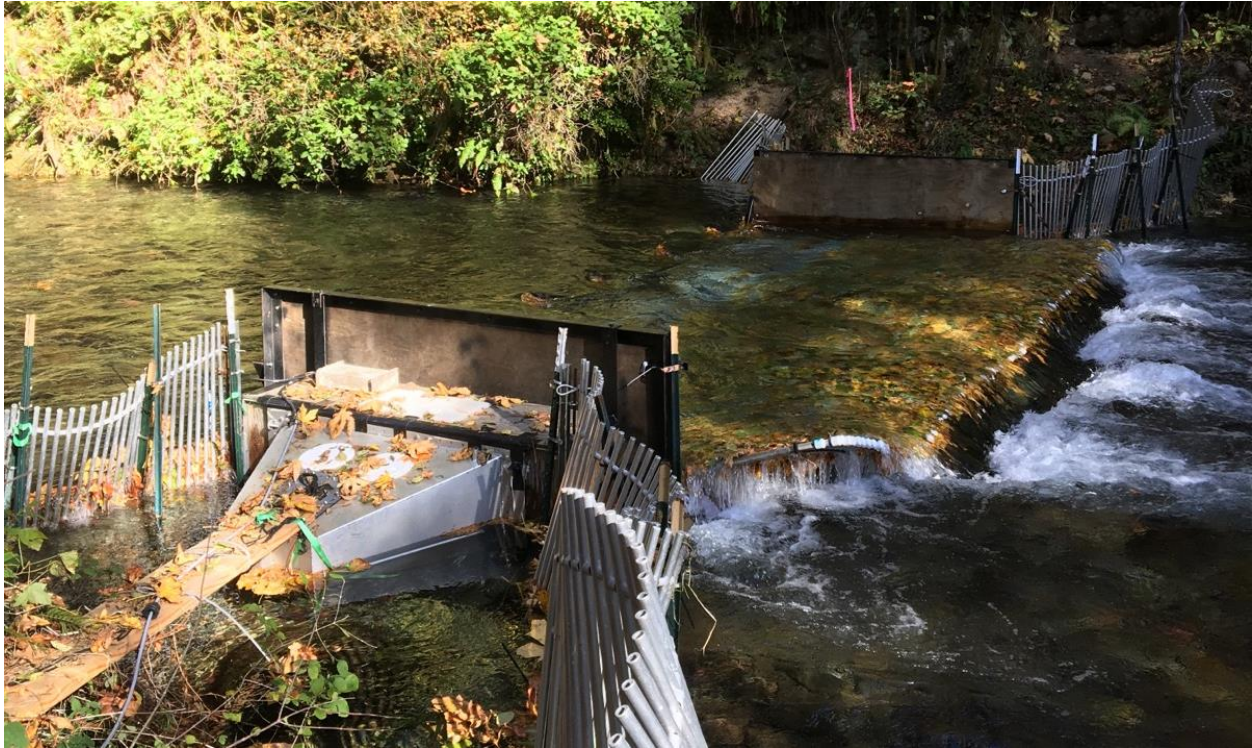
Figure 6. Example of high debris levels and elevated streamflows in early November 2020 at the Cougar Creek video weir.
