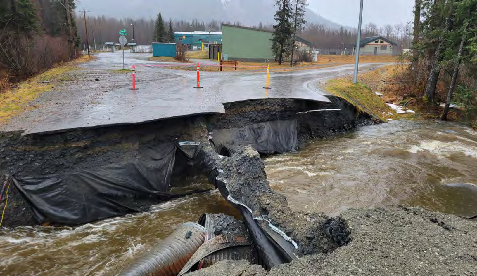
Photo: Heavy rains, flooding, and a washed out culvert in Girdwood, October 2021. (Dave Leval, KTUU)
