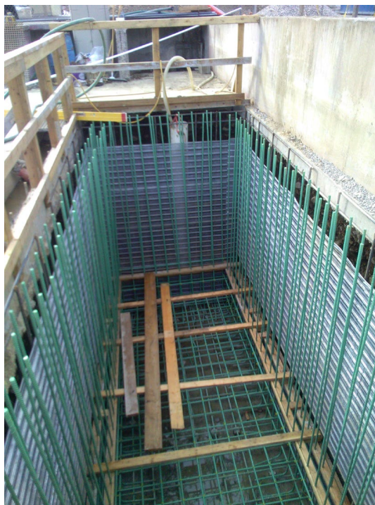
Rebar in flume-sump prior to pouring concrete. USFWS Photo—Jason Ilgen
