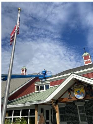
A four-person Great American Outdoor Act Deferred Maintenance Strike Team spent two weeks working on the exterior of the Nulhegan Basin Office/ Visitor Center. The maintenance crew rebuilt the cupolas, replaced most of the trim along the roof line/windows, replaced rotten clapboards and re-flashed areas that required attention. A big thank you to the New Hampshire crew for their support of the Conte Refuge.
