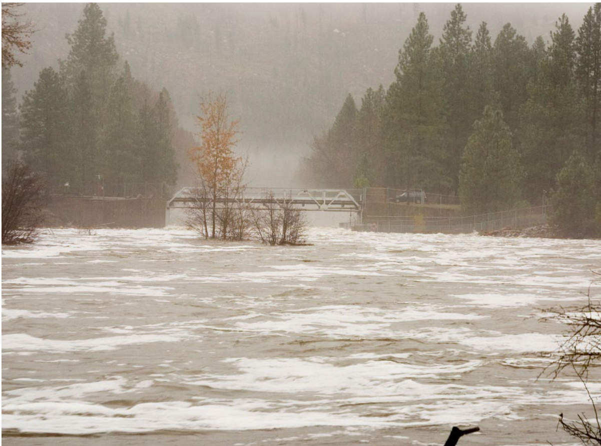
Figure E1. High water of Icicle Creek on November 6, 2006 (~14,700 cfs) looking upstream towards the bypass canal and dam (under and behind the bridge). The cyclone fence next to the fish ladder is visible to the right of the bridge below the parked vehicle. The water level downstream of the dam is nearly even with the water level in the canal upstream of the dam. See also Figures E2, E3, and E4.
