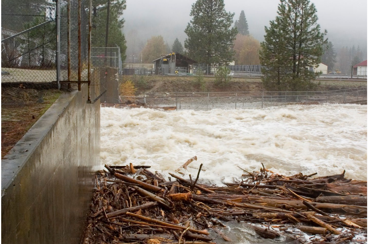
Figure E3. Icicle Creek in the tailrace area immediately downstream from the canal dam looking towards the fish ladder (marked by the cyclone fence) and spawning shed during the high water event of November 6, 2006. The superstructure of the bridge over the dam is visible near the upper-left corner of the photograph (compare to Figure E1).
