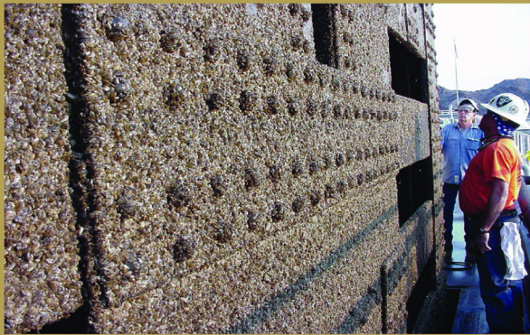
The surface of a normally underwater part of the Davis Dam in Nevada, just downstream from the Hoover Dam on the Colorado River, covered with invasive quagga mussels.
