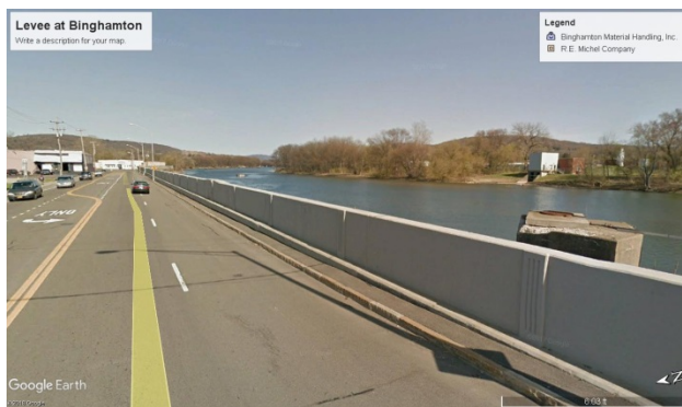
Figure 1. Floodwall along Susquehanna River at Binghamton (Google Earth)
