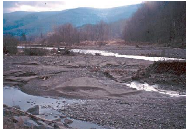
This stream segment was over-widened with bulldozers to make room for floodwater (photo by NY City Department of Environmental Protection).
