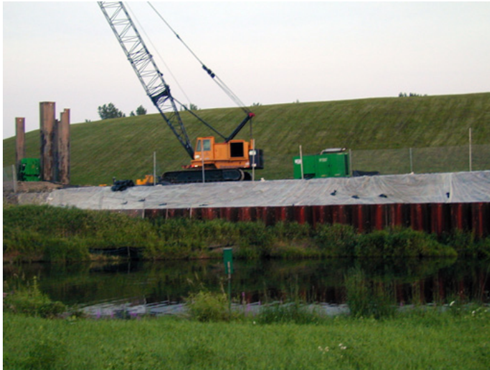
Turtle Cove prior to cleanup of PCB-contaminated sediments. The unlined 12-acre GM Landfill was capped with clay and seeded with grass.
