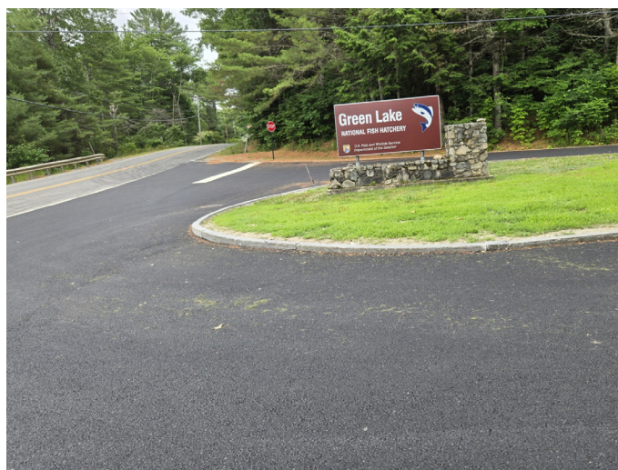
Green Lake NFH Entrance Road after a Fresh Coat of Asphalt. Source: Rich Yee, FWS
