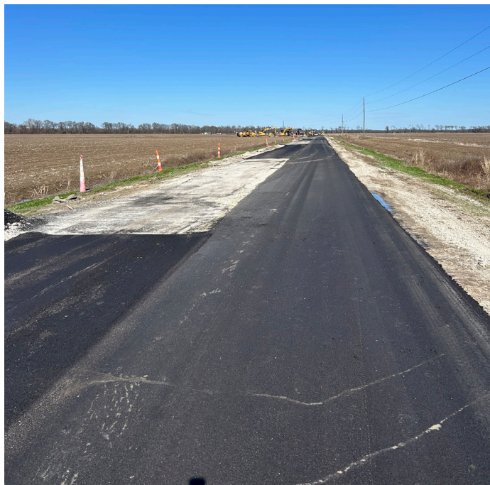
Completed Section of Asphalt Repair as part of the Surface Preservation Project at Tensas River NWR in Louisiana. Source: DOT Construction, INC.
