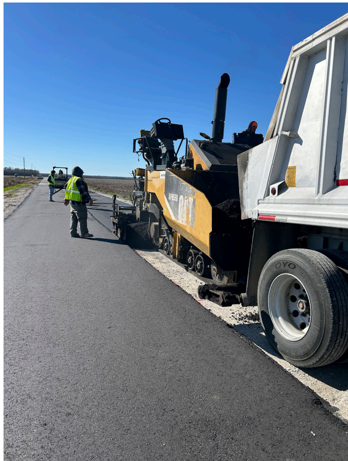
Roadway Paving as part of the Surface Preservation Project at Tensas River NWR in Louisiana. Source: DOT Construction, INC.
