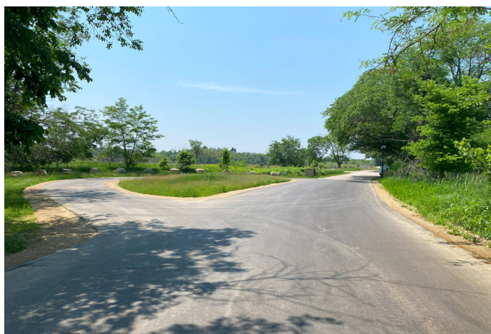
Entrance Road Gate Turnaround (Post Project) at Trempealeau NWR. Source: FWS
