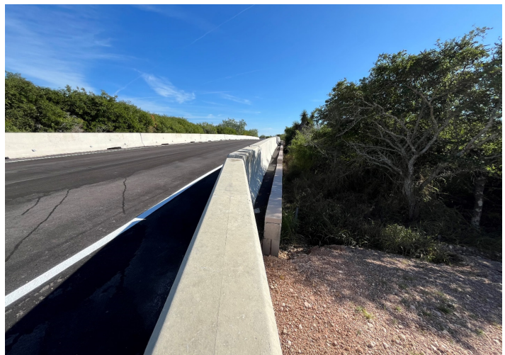
Jersey Barriers and Wing Walls to Protect Wildlife and Visitors at Laguna Atascosa NWR. Source: Nate Begay, FWS
