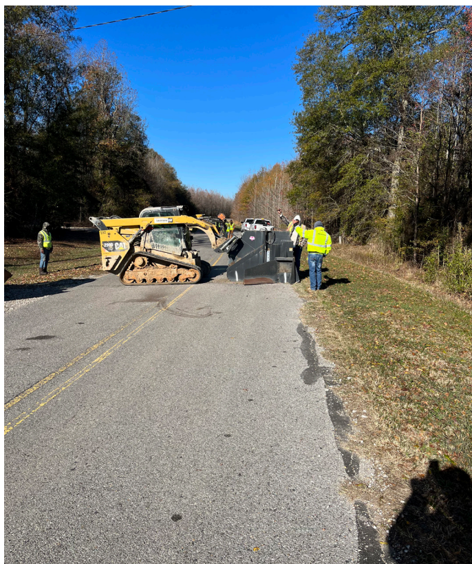
Beginning Asphalt Rehabilitation as part of the Surface Preservation Project at Tensas River NWR in Louisiana. Source: DOT Construction, INC.
