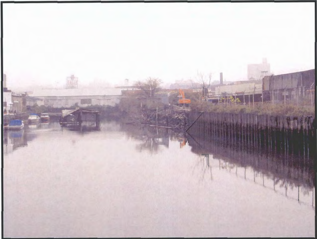
Plate 3.5. Gowanus Canal Assessment of Eligibility: View southeast of the 6th Street basin. A steel sheetpile bulkhead is seen at the right of the view, with a collapsing timber bulkhead visible beyond (center right of view). An intact timber bulkhead (center left of view) and a steel bulkhead (left) can also be seen (Photographer: Thomas Flagg , November 2003) [Source: Raber Associates].
