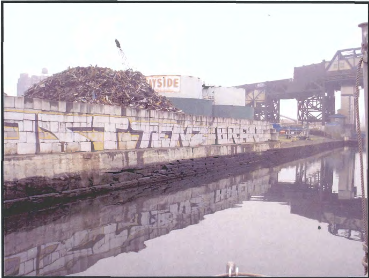
Plate 3.14. Gowanus Canal Assessment of Eligibility: View northeast near the 11th Street basin showing concrete additions to the cribwork bulkhead face (left) and new timber face on cribwork bulkhead (right). The New York Transit Authority trestle is visible in the background (Photographer: Thomas Flagg , November 2003) [Source: Raber Associates].
