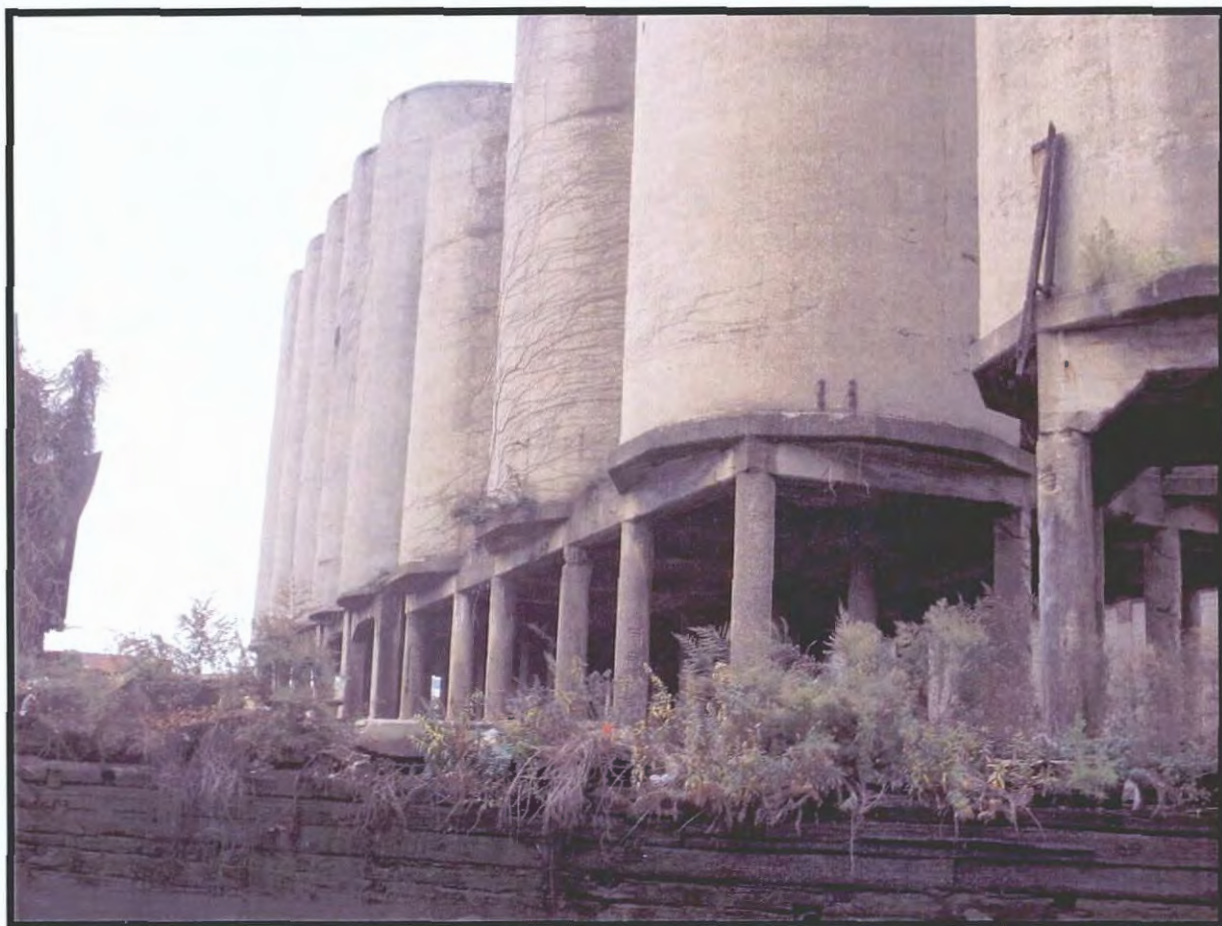
Plate 3.21. Gowanus Canal Assessment of Eligibility: View southwest of Burns Bros. Coal Pockets and timber cribwork bulkhead near the head of the 4th Street Basin (Photographer: Thomas Flagg, November 2003) [Source: Raber Associates].
