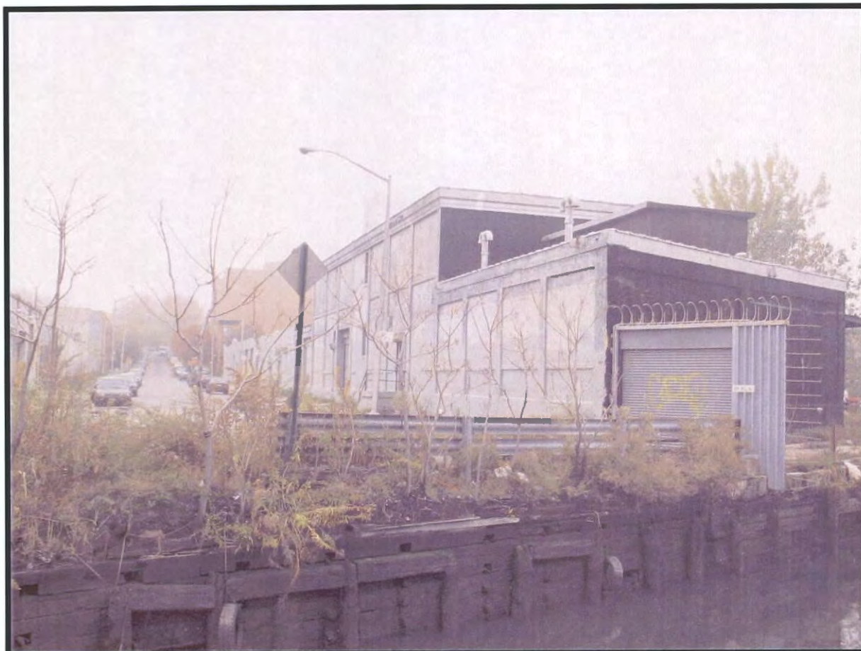
Plate 3.9. Gowanus Canal Assessment of Eligibility: View northwest of the intact timber crib-work bulkhead at the end of 1st Street, with a 1916 concrete oil terminal structure (Photographer: Thomas Flagg, November 2003) [Source: Raber Associates].
