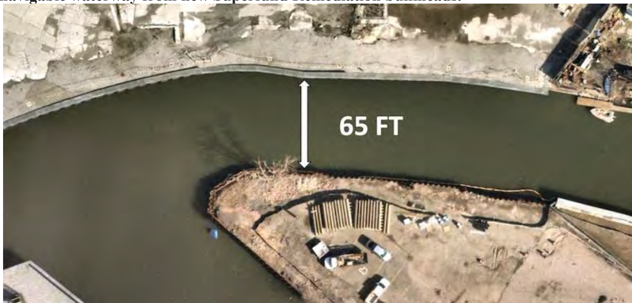
2024 - 8 March Nearmap aerial of bulkheads expanded into Canal at 5 th Street (Public Place)
