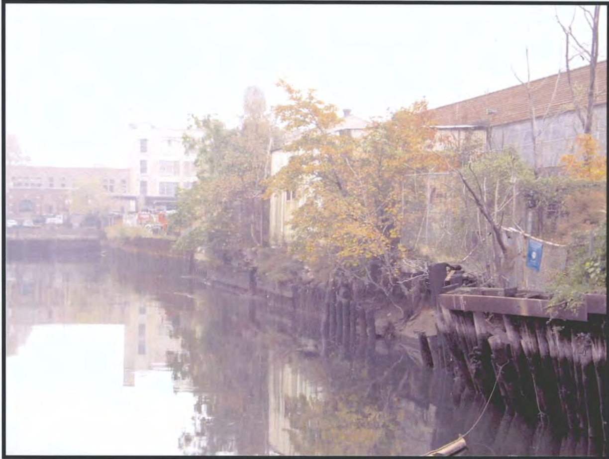
Plate 3.10. Gowanus Canal Assessment of Eligibility: View northeast towards the end of the canal, with timber sheetpile (right) and steel sheetpile (left center) bulkheads, and concrete bulkhead at the end of the canal (left) (Photographer: Thomas Flagg, November 2003) [Source: Raber Associates].
