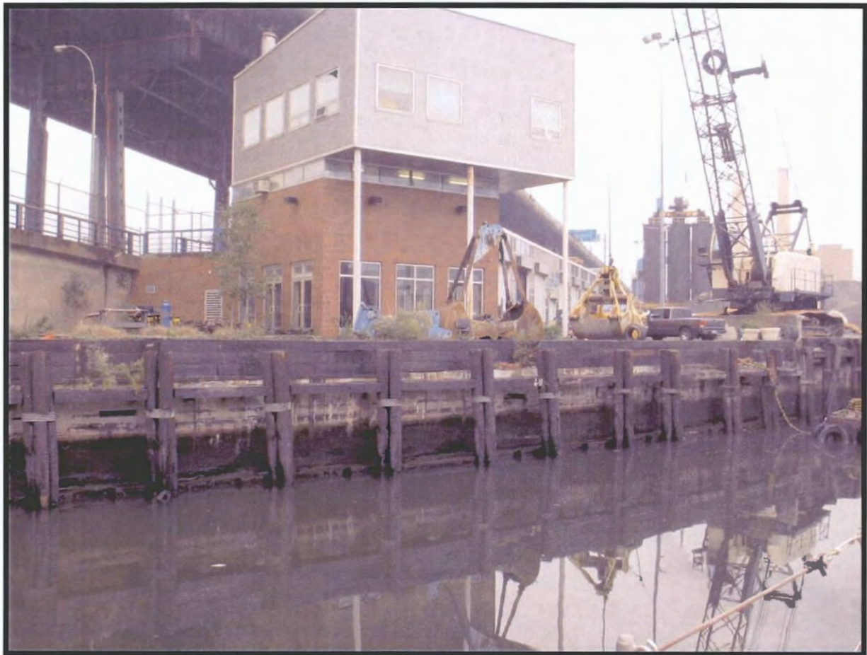
Plate 3.1. Gowanus Canal Assessment of Eligibility: View south of recent bulkhead at 14th Street, with concrete face above possible cribwork cut off at the mean low water mark (Photographer: Thomas Flagg, November 2003).
