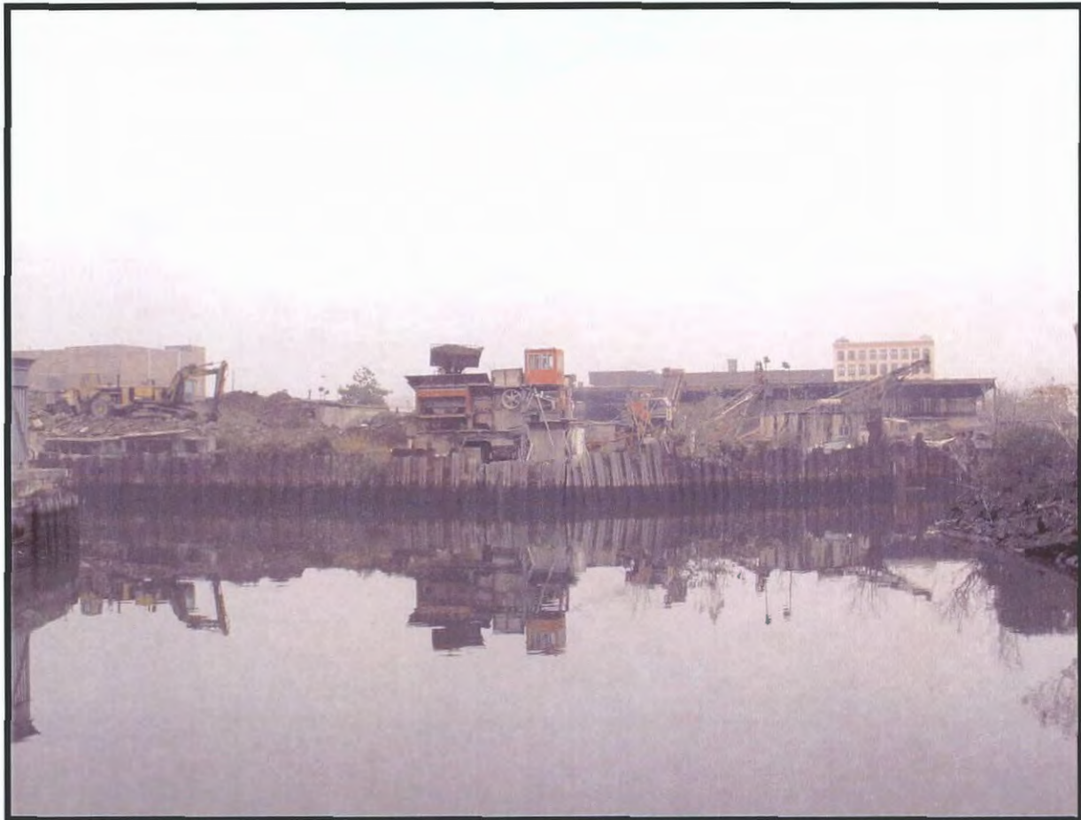
Plate 3.7. Gowanus Canal Assessment of Eligibility: View east of steel sheetpile bulkhead and crushing plant at the junction of the main canal (left of view) and the 4th Street Basin (Photographer: Thomas Flagg , November 2003) [Source: Raber Associates].
