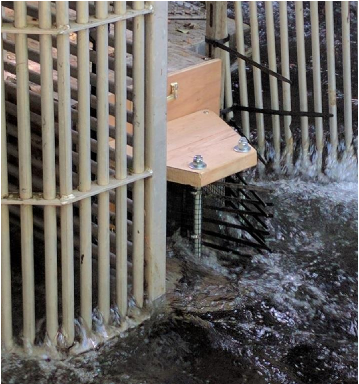
Figure 4. Exclusion gate for video chute.
