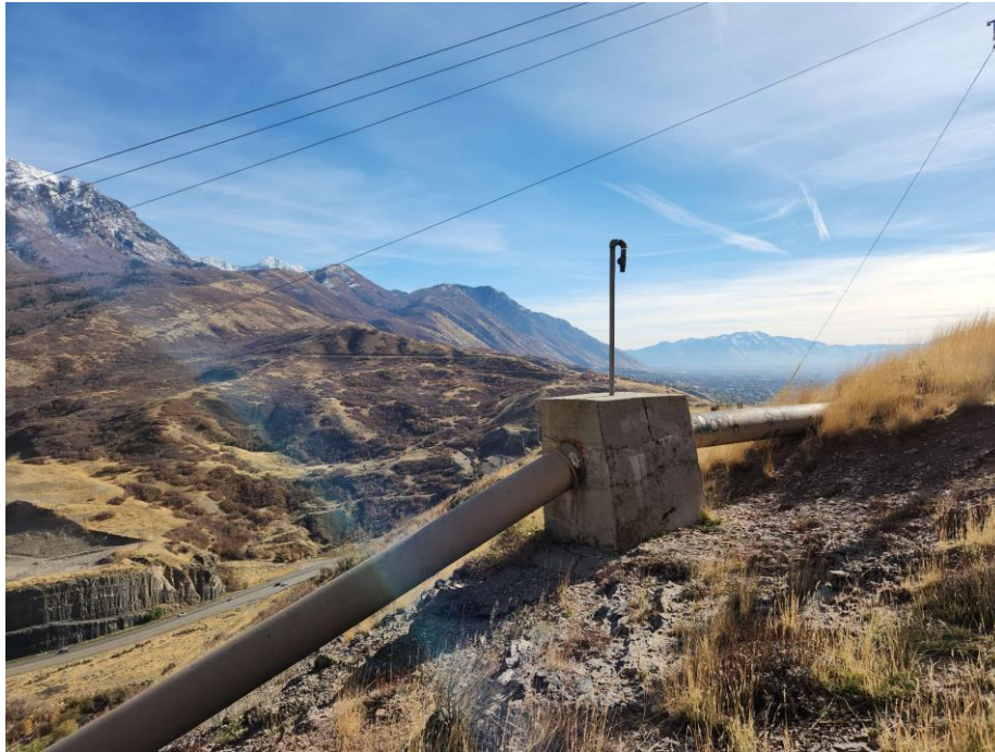
Figure 9. Overview facing southeast showing IO-02 potentially historic pipeline. Photo taken November 13, 2024.
