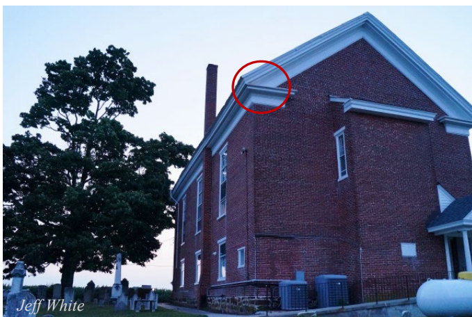
Figure 26 (left) and 27 (right). Keep in mind that potential bat access points may not be obvious or even visible from the ground. In this example, an emergence survey reveals bats exiting through a gap in the trim board above the second story of a church. Inside, this is the far corner of the attic floor.
