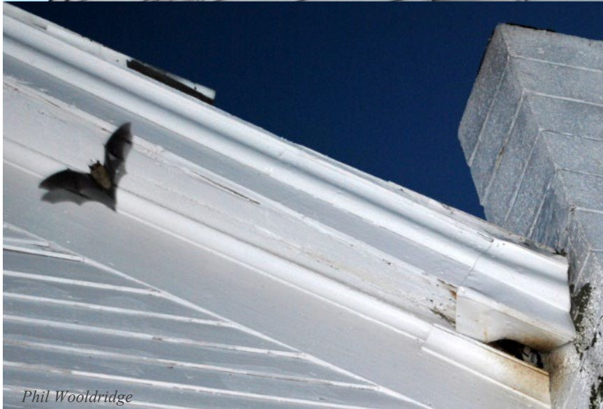
Figure 25. A bat photographed emerging at dusk from the eave of a church. Staining is visible around the entry/exit point where the eave meets the chimney. The eave had rotted at this junction, and the flashing used to cover it is warped from bats coming and going over the years.
