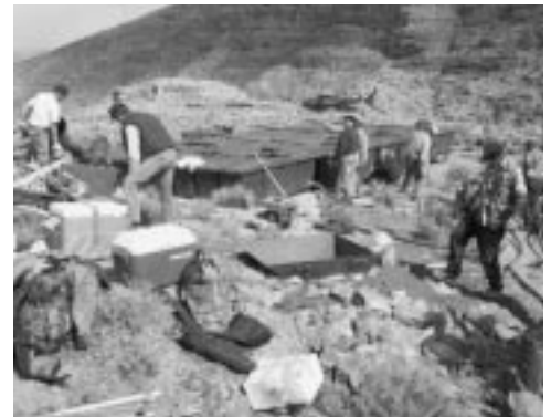
Rain catcher. A 45-foot by 70-foot steel apron feeds infrequent rains to these four 1,800-gallon tanks. Rock will be cemented around the water trough (center) to bring it up to ground level. FWS photo: Dick Birger.
