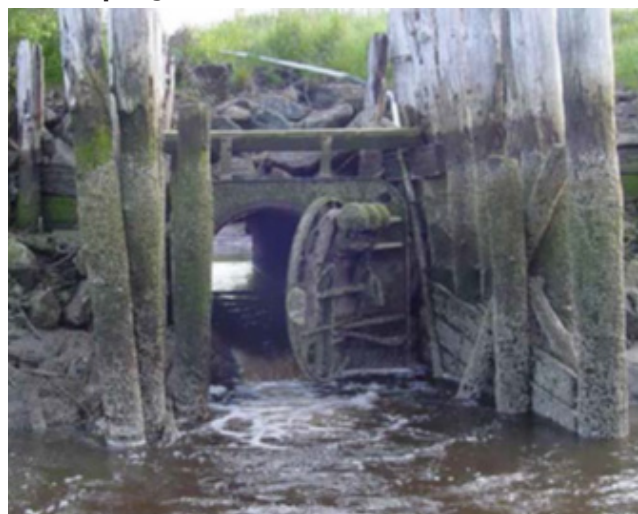
Figure 11. Fahys Creek tide gate during mid-ebb tide in late spring, 2010
