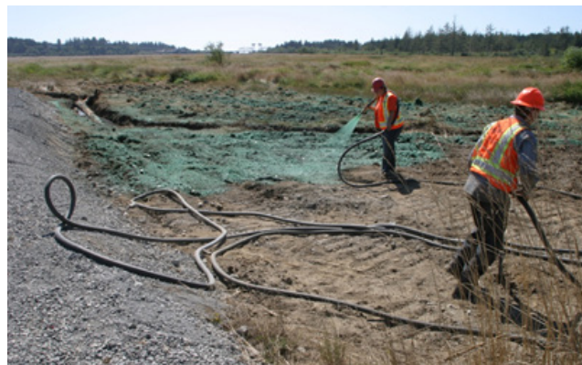
Figure 35. Applying hydro-seed mixture to disturbed soils near the elevated gravel path into the marsh
